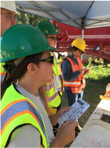
Field day attendees observing drilling activities and preparing to log a boring. Photo courtesy of Linda Hensel.
